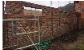
THE WALLS ARE GOING UP!
